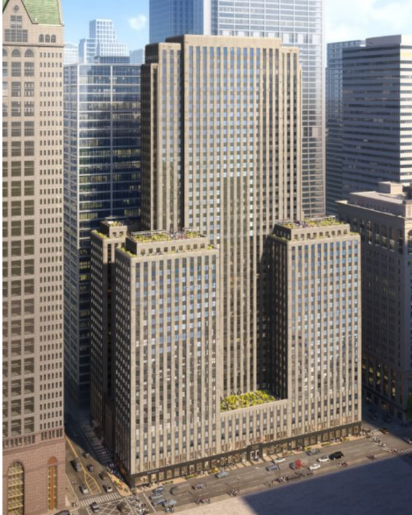
Office-to-Residential Conversion Project
